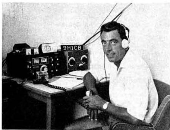
Ken Randall, 9H1CB, seated at the rig in his cabin on top of St Angelo, 200ft above Grand Harbour, Malta. The cabinet on the right contains a Z-match for the 40/80m trap dipole, and the small Perspex box covers the paddle of an electronic keyer which was designed by 9H1AZ.
